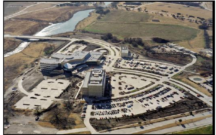
Children's Medical Center at Legacy Under Construction - Spring of 2008
